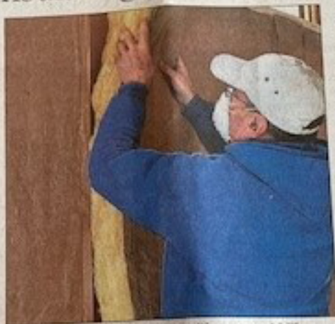
Installing insulation in wall cavities can cut bills
